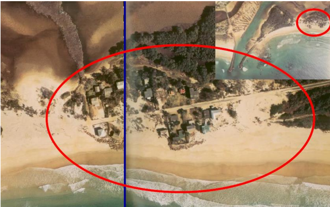
Figure 5. The destruction of Sheltering Palms village to the north of the entrance breakwaters on the Brunswick River
