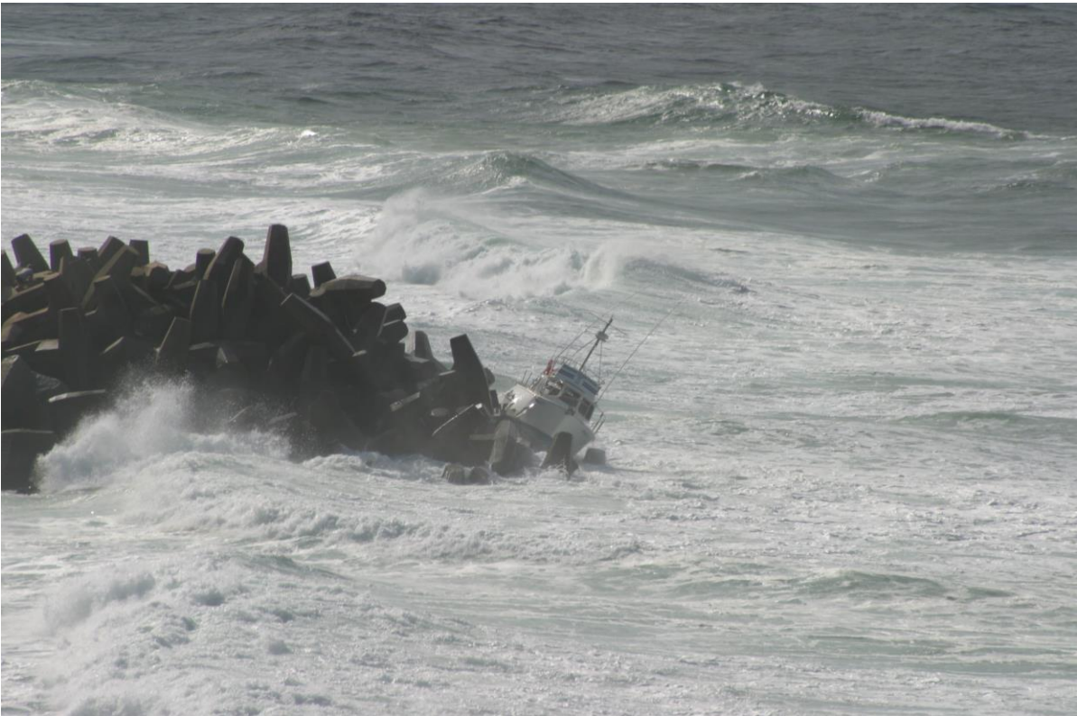
Figure 11. Charter boat smashed on the end of the Narooma Breakwater (Photo Batemans Bay Post). Since 1970 there have been more than 11 deaths and 100 rescued.
