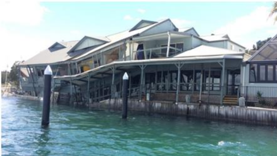
Figure 9. At Lake Macquarie, the collapse of a Swansea Channel foreshore building comprising restaurant, offices and residences on 8 February 2016 (Photo: Fire & Rescue NSW).
