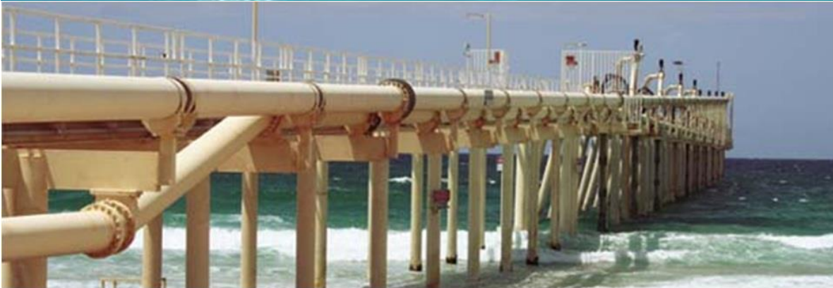
Figure 2. Tweed River entrance and sand-bypassing system comprising trestle, sand pumps and pipelines (©Tweed River Entrance Sand Bypassing Project (TRESBP))
