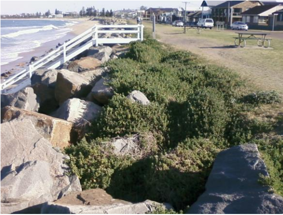
Figure 10. Left: Rock revetment to protect Mitchell Street. Right: Severe erosion north of the rock revetment
