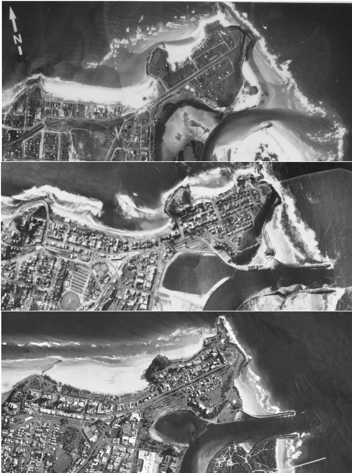
Figure 1. Top: Tweed River entrance in 1935 prior to breakwater extension. Centre: Tweed River entrance in 1967 following breakwater extension. Note improvements to channel navigation and the depletion of Coolangatta Beach. Bottom: Tweed River entrance in 2004 following installation of sand bypassing system. Note accretion of Coolangatta Beach. (from Ackworth & Lawson, 2011)
