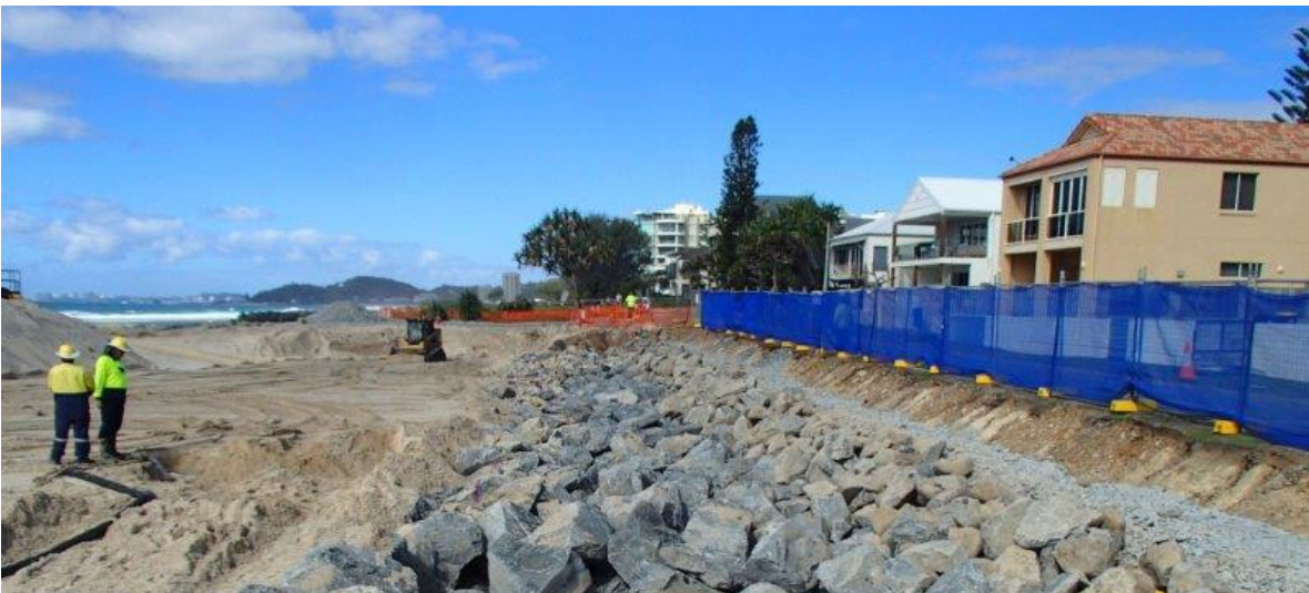
Figure 3. Revetment under construction, Palm Beach, Gold Coast
